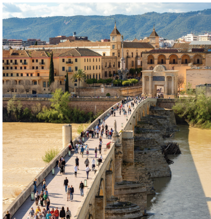
The Roman Bridge of Cordoba
