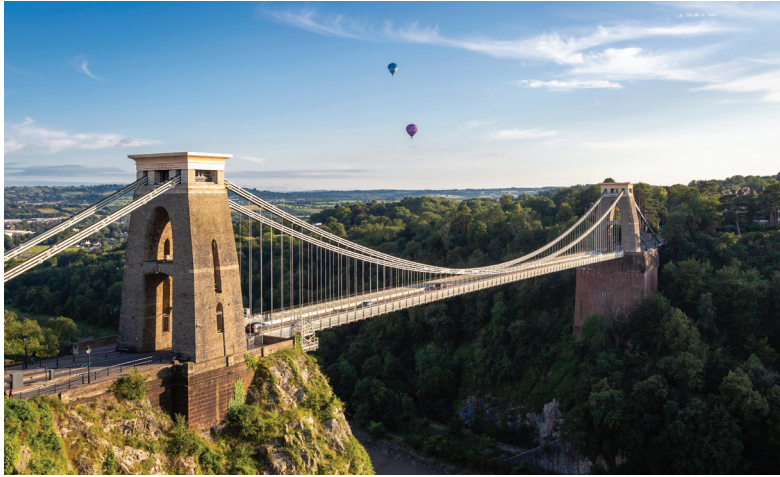
The Clifton Suspension Bridge
